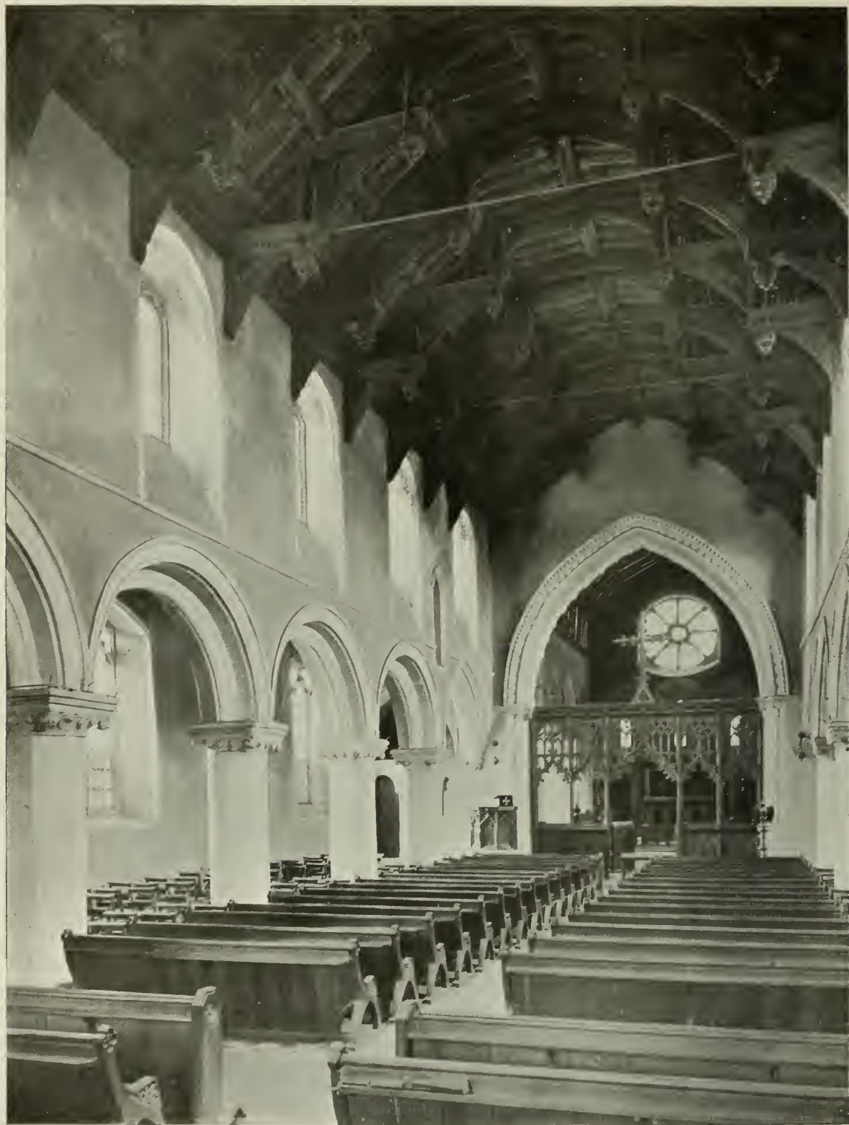
CASTLE HEDINGHAM: PARISH CHURCH OF ST. NICHOLAS. North Arcade, c. 1180 and 14th-century; roof of Nave, early 16th-century.
